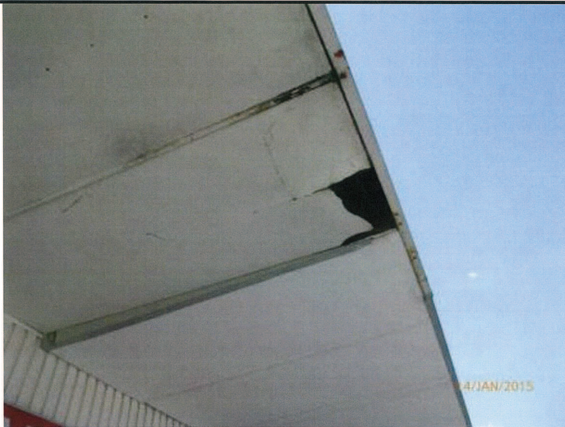
I: 26-30 Good Street – awning
